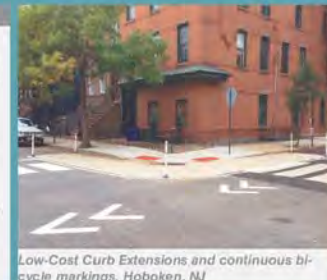
Low-Cost Curb Extensions and continuous bicycle markings, Hoboken, NJ
